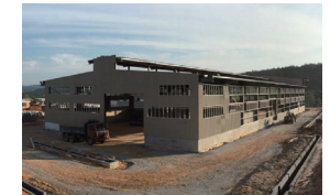
Under construction (as of Feb 2017)
