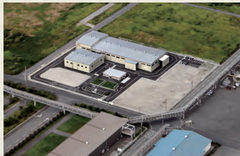
The AMITA Kitakyushu Resource Recycling Plant in Kitakyushu Eco-Town, where various recycling industries are concentrated
